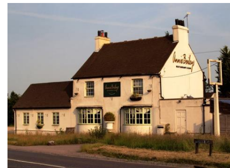
Annie Baileys, demolished for HS2
